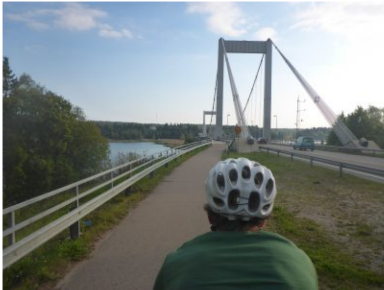
First bridge onto the Archipelago
