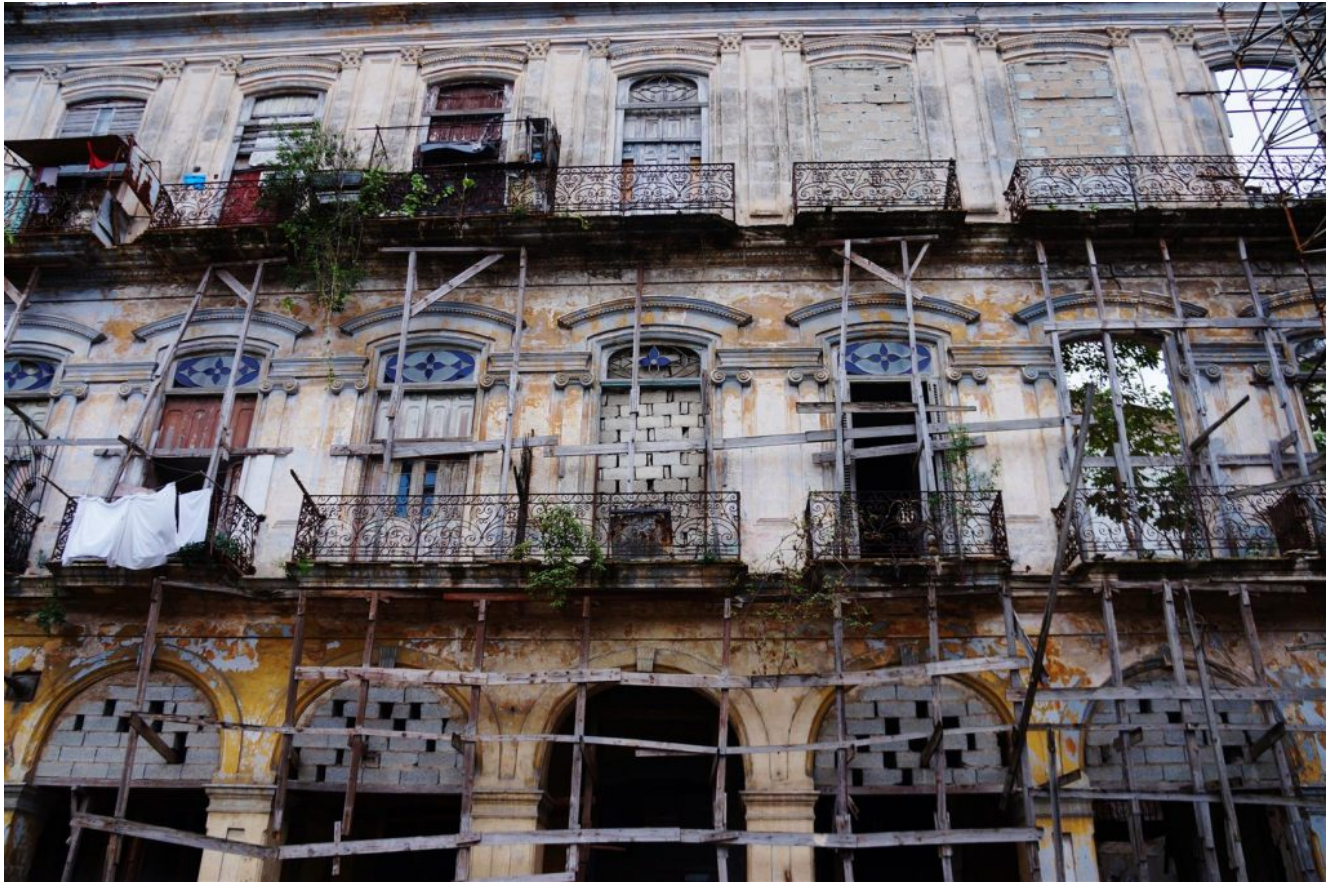
Scaffolding in Havana
